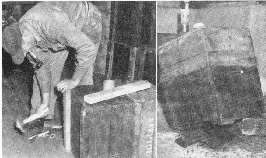
The above photo, left, shows Marshall Steele of the Oil House replacing a defective cleat on an acid carboy. As is true of many containers, carboys go bad at the bottom first, as illustrated in the photograph on the right.
